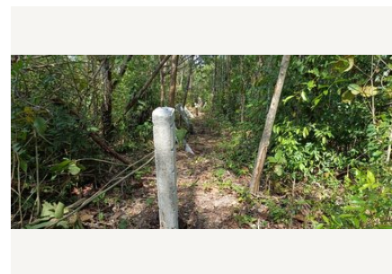
Post for right-of-way demarcation.
