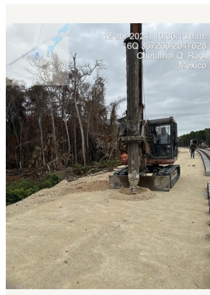
Drilling with crawler-mounted equipment.
