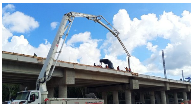
Superstructure casting with concrete pumping.
